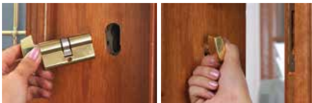
D. Put in a new profile cylinder.
