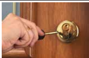
C. Remove the screws and take off the internal cover.
