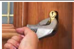
D. Tighten up with a switch wrench and swing it. (cylinder is exposed by at least 10mm).
