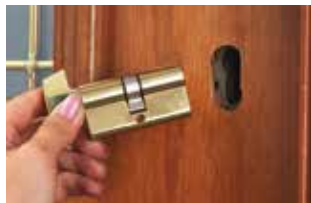
E. The profile cylinder can be broken off easily.
